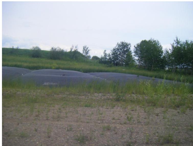
**Figure 4.7: Geotubes for Sludge Dewatering**
