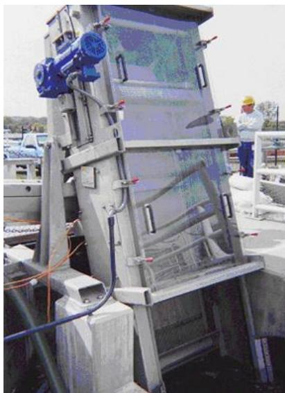
**Figure 6.1: Typical 6 mm Bar Screen (Photo Courtesy of Headworks)**
