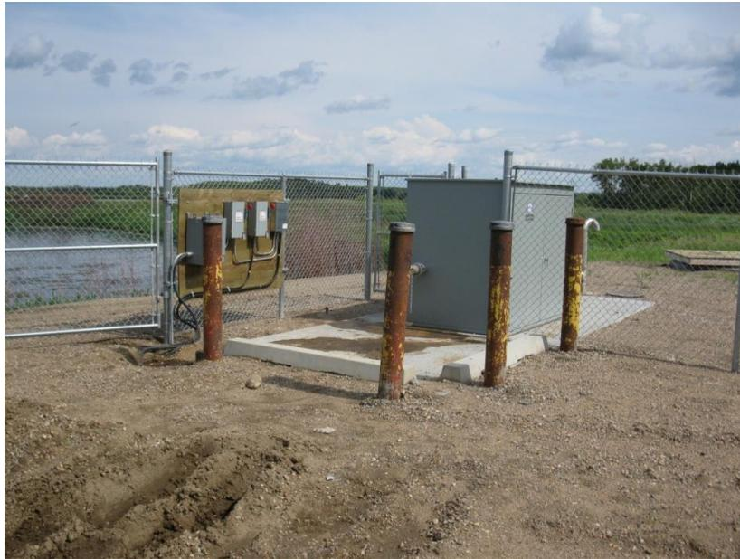
**Figure 4.8: Septage Receiving Station**
