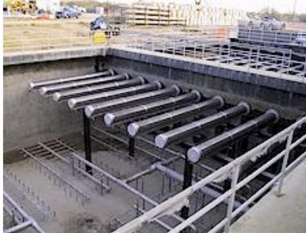
**Figure 6.15: A Typical MBBR Basin Installation with No Media Installed (Photo Courtesy of Veolia)**
